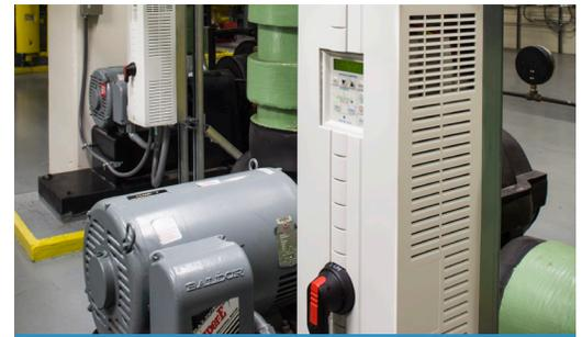
VFDs installed on chilled water pumps paid for themselves in energy savings in about a year.
