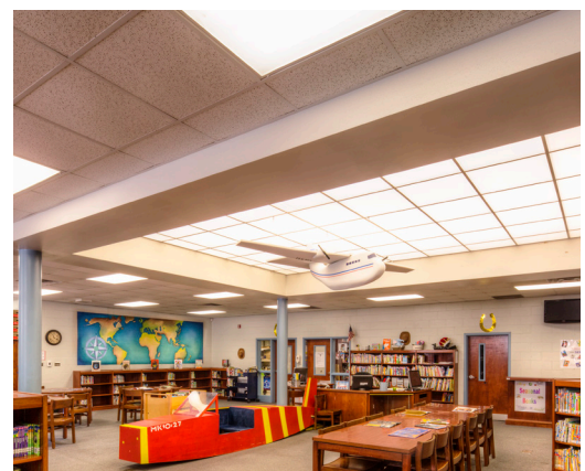
Brighter, more consistent lighting in the library at Temple Elementary makes for a better learning environment.
